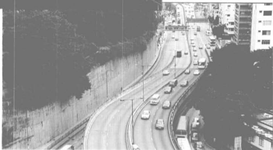
▶ 新公主道天桥, 1989年开通 (The new Princess Margaret Road Flyover)
