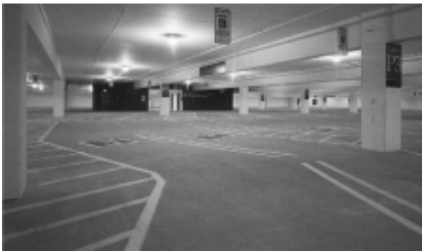
FIGURE 1.1 One-way reinforced concrete floor slab with monolithic supporting beams. ( Portland Cement Association. )
