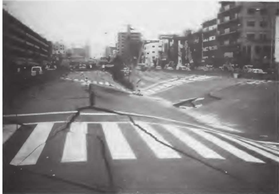
Fig. 1.3 Surface subsidence due to the damages of subway station
