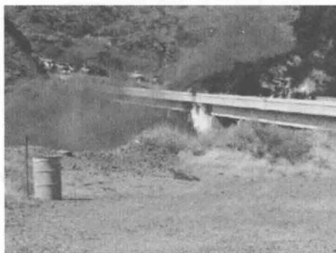
图 1-3 Bill Williams River Bridge(2006)
