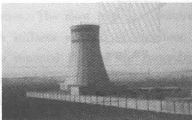
(c) petrochemical container engineering
