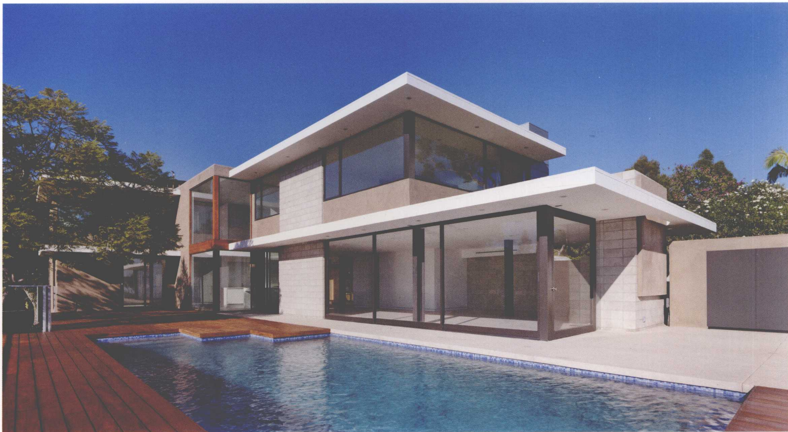
General view 建筑外观
