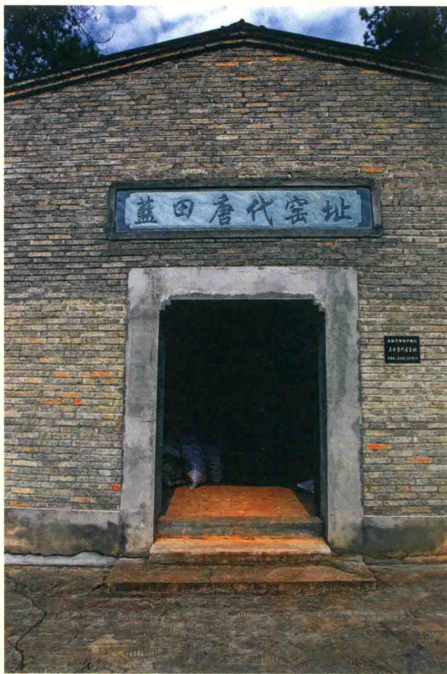
兰田龙窑保护房外景 The Protection House of the Dragon kiln in Lan tian
