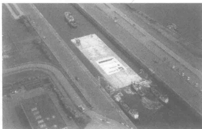
图6 当沉管浮运了70km之后,在外海上将穿过艾默伊登水闸的管节 (Element passing the locks of Ijmuiden after towing 70 km over open sea)
