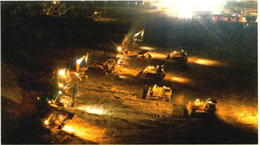
An aerial view of the Huoshenshan Hospital site, Wuhan. (Photo by Xiao Yijiu, Xinhua News Agency)
