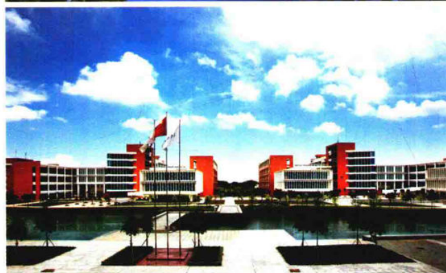
广州大学城华南理工大学新校区总体规划 / 162 PLANNING OF NEW CAMPUS OF SOUTH CHINA UNIVERSITY OF TECHNOLOGY IN GUANGZHOU HIGHER EDUCATION MEGA CENTER
