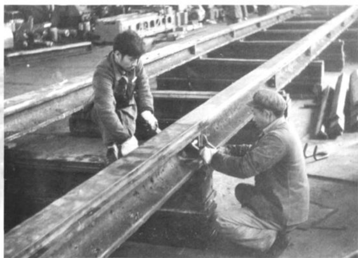
建厂初期为龚嘴电站拼装主轨
