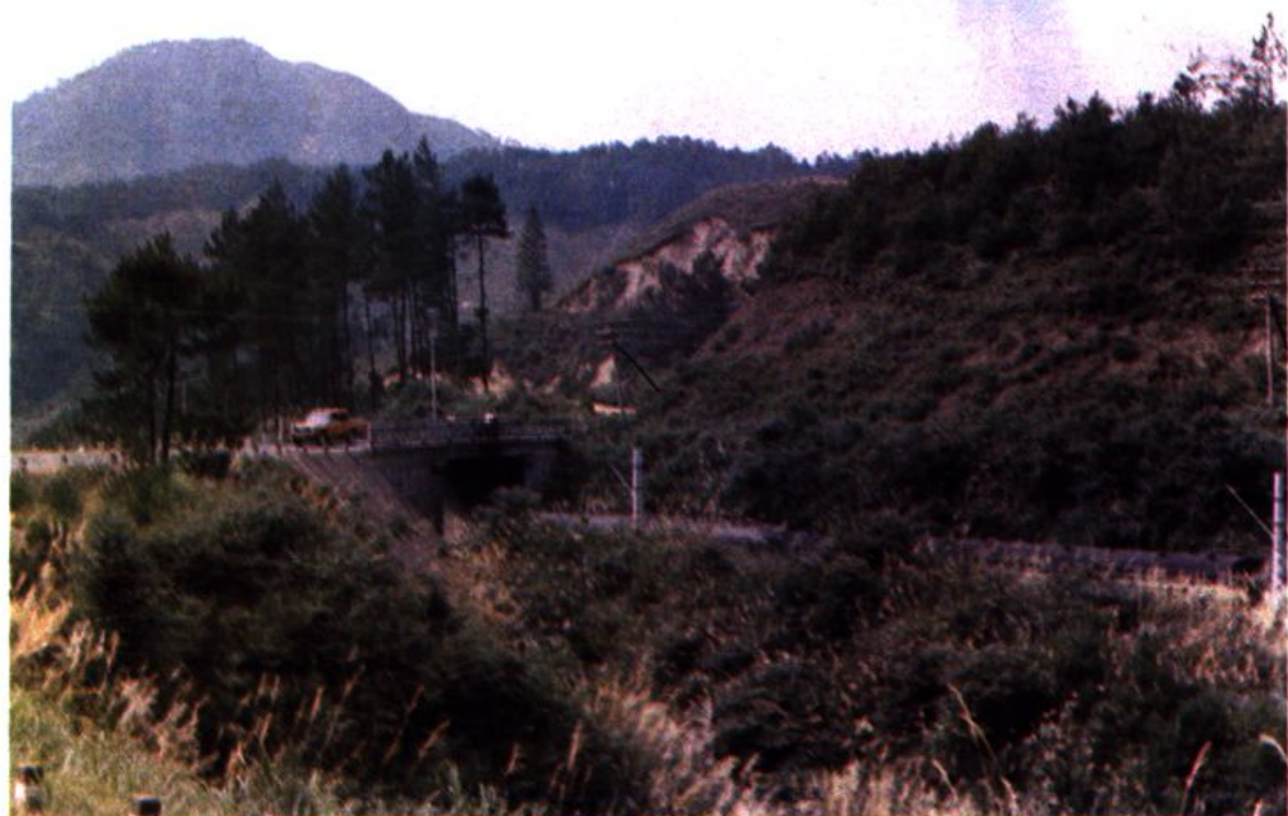
“316”线公路立交桥(467 k +706)
