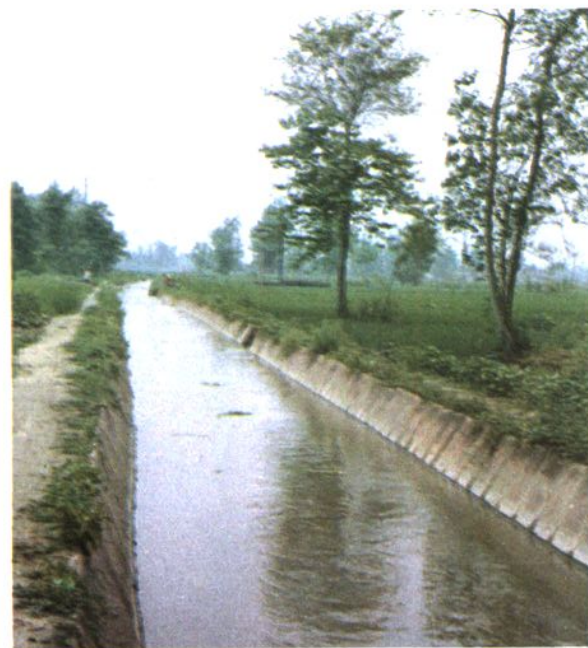
粉后堰浆砌支渠
