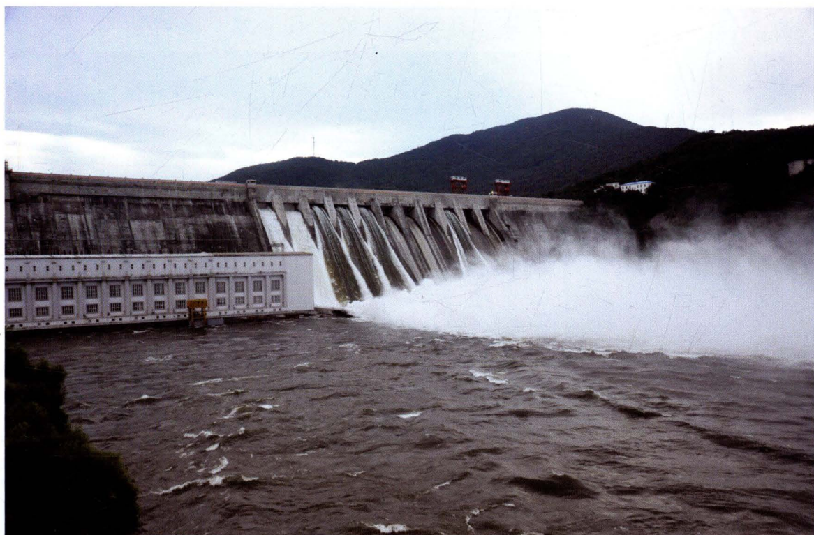
丰满发电厂大坝泻洪
