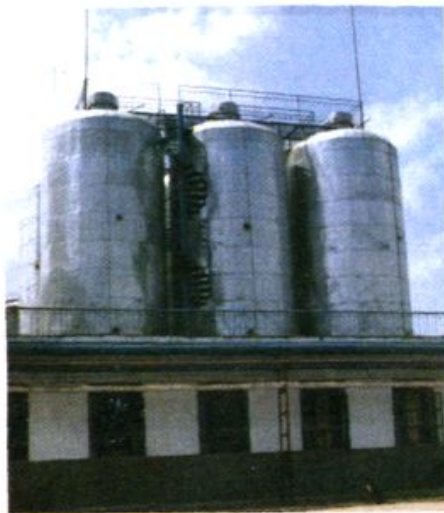
新扩建的露天锥形发酵罐▲
