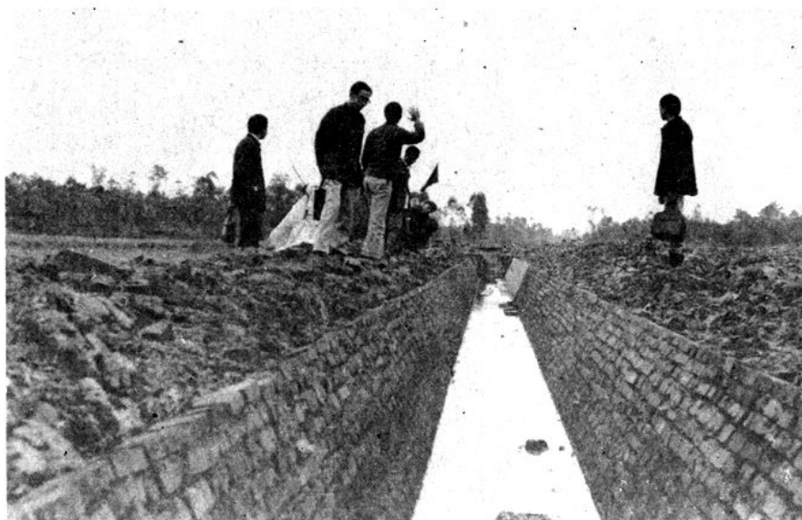
坝区开沟排湿
