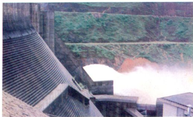
△峰头大坝背水坡砌筑工艺
