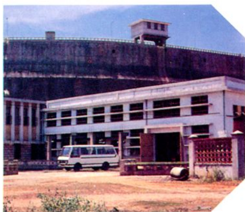
峰头水电站厂房
