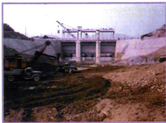
增建2号副坝泄洪闸
