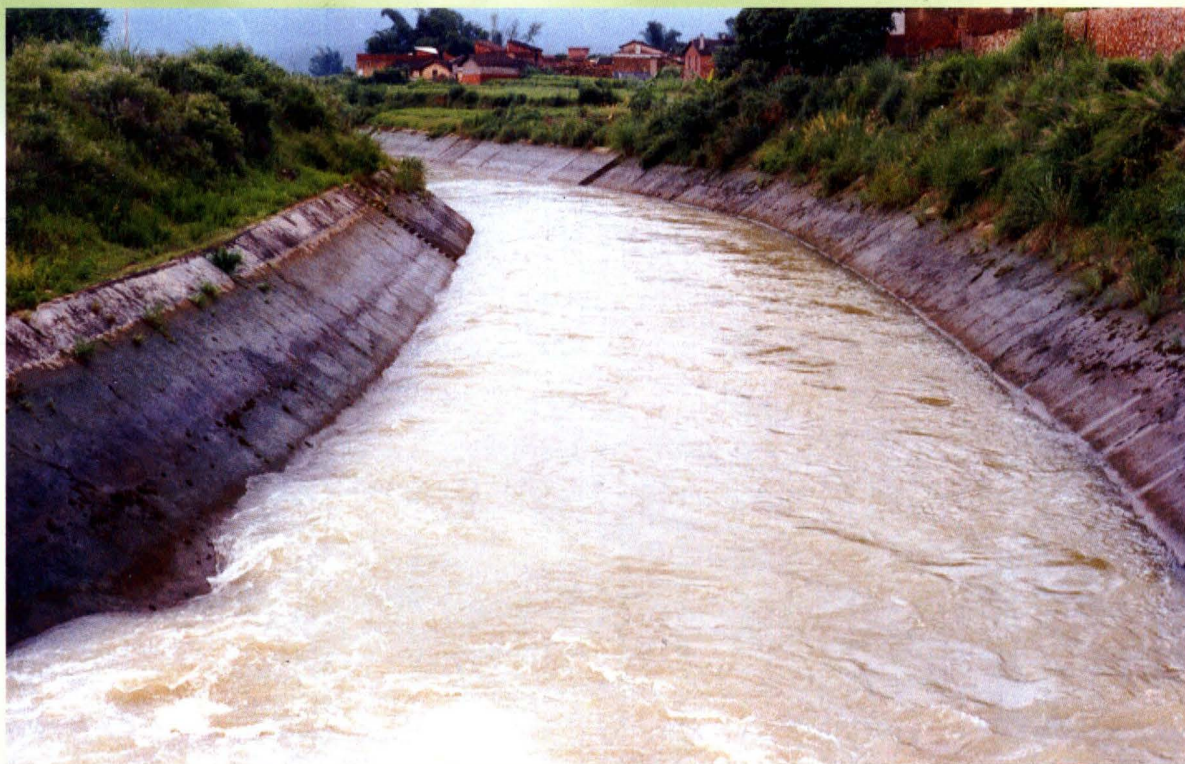
蕉岭县长潭干渠
