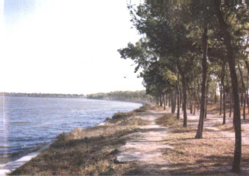
蓟运河弯道护坡
