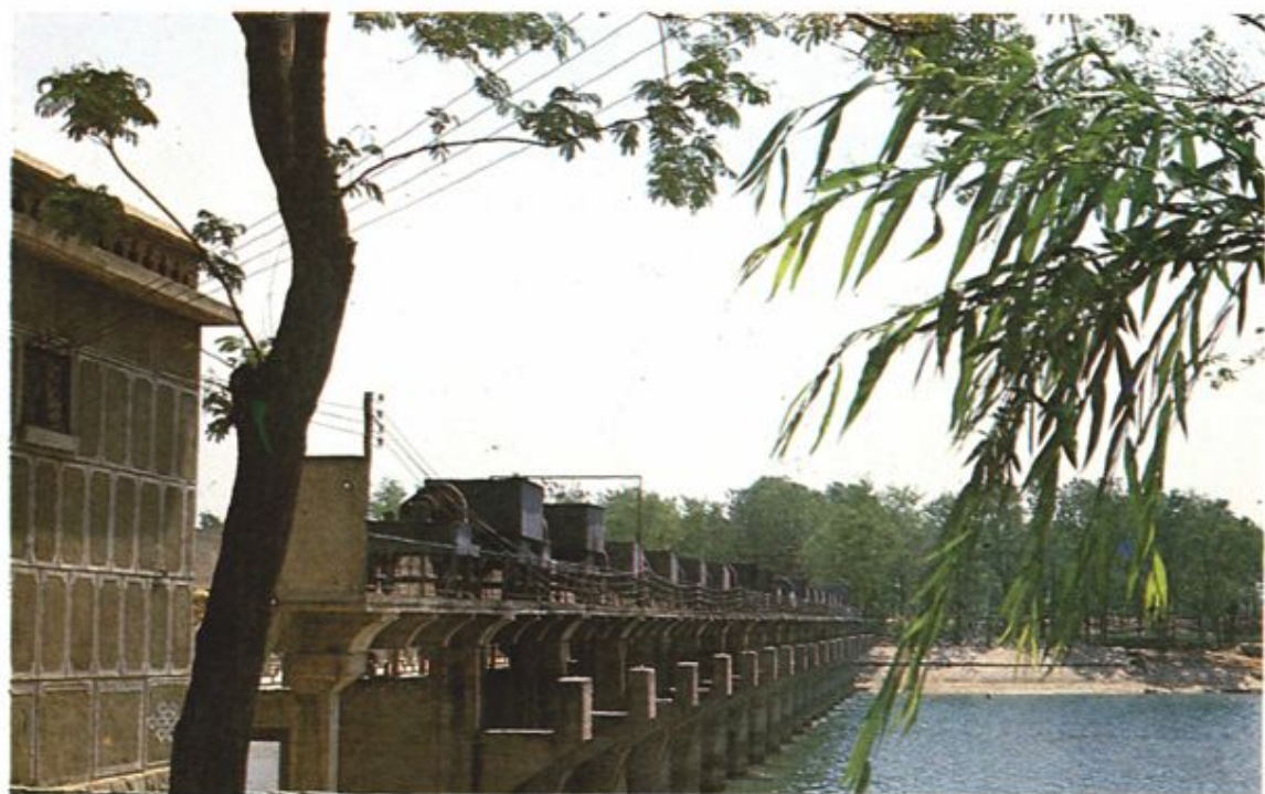
徒骇河樊家桥栏河闸
