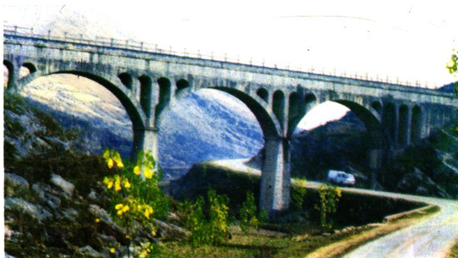
跳墩石拱渡槽( L=86M^3Q=5M^3/s )
