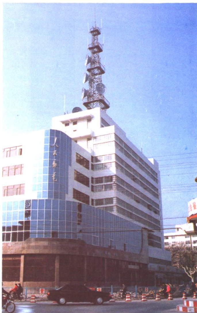
宿县地区邮电大楼
