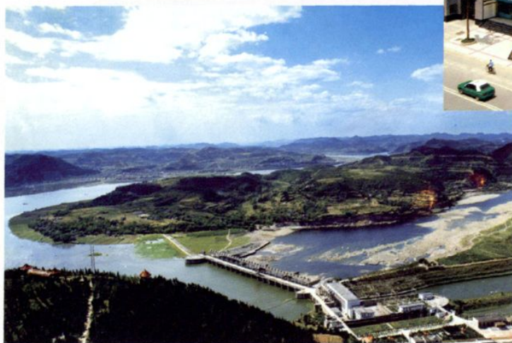
螺丝池水电厂全貌
