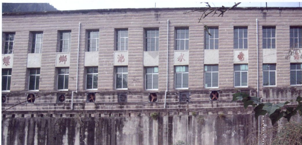
螺丝池水电厂一车间厂房
