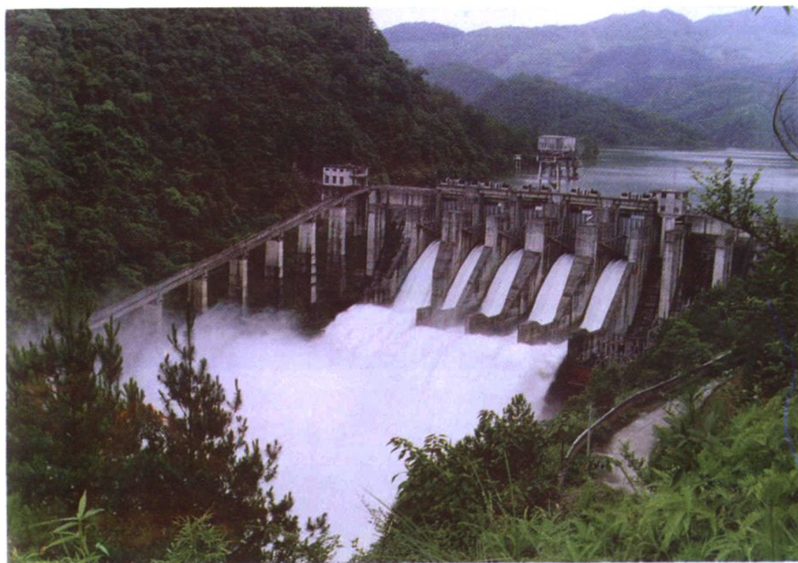
池潭水电厂宽缝重力坝
