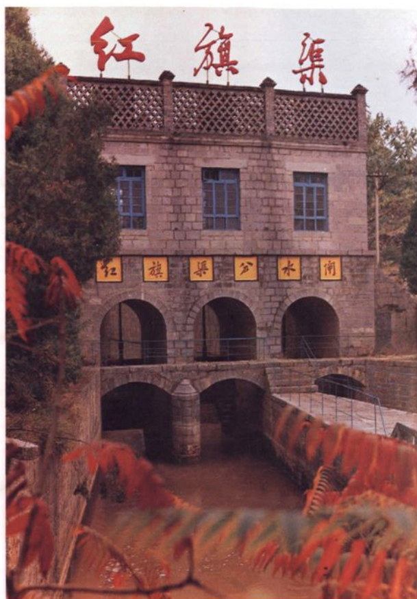
红旗渠总干渠分水闸
