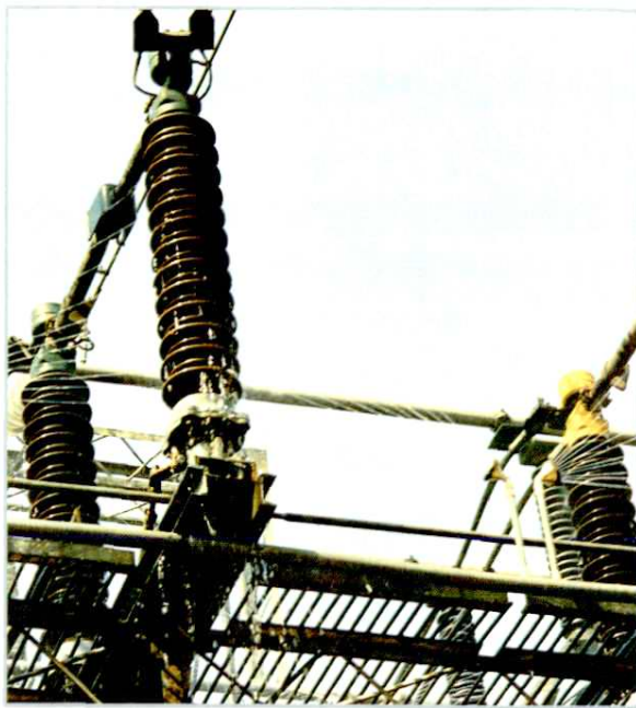
330千伏南郊变电站带电水冲洗
