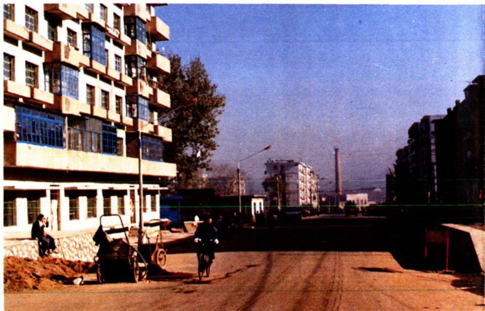
新擴建公路 Widened road
