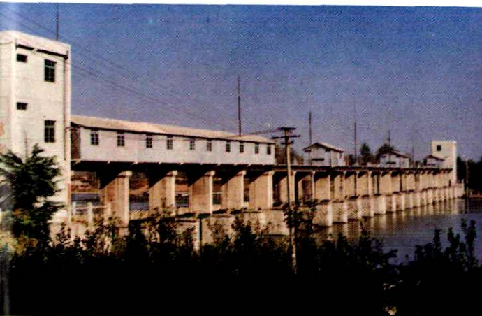
复兴河节制闸
