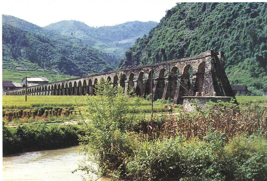
岜暮乡板么引水渡槽
