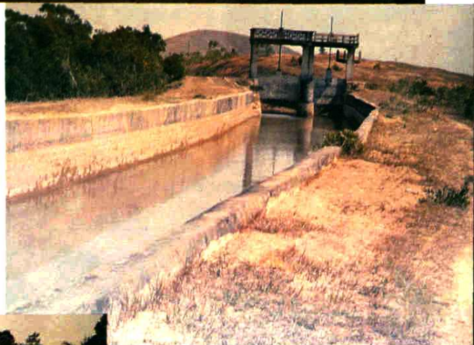
总干渠双金围节制闸
