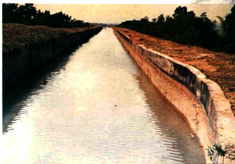
双金围段砌石槽
