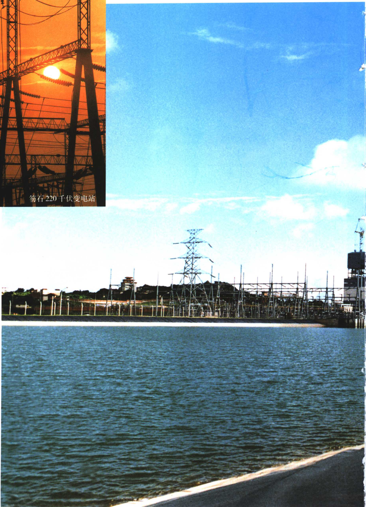
湄洲湾火电厂
