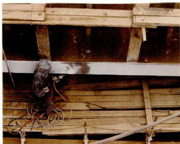
闸门除锈喷锌
