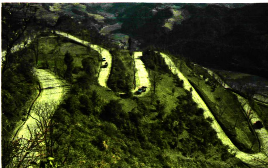
▶ 永万线凉亭坳盘山公路
