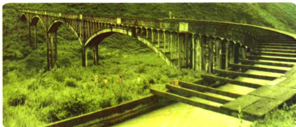
宜昌市东风渠灌区蜘蛛洞双曲拱渡槽
