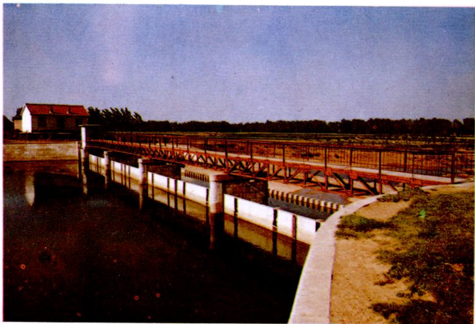
胶河鸾庄拦河闸
