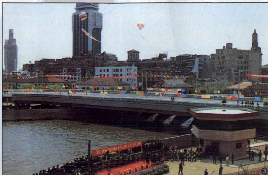
吴淞路闸桥 Wusong Road Barrier Bridge
