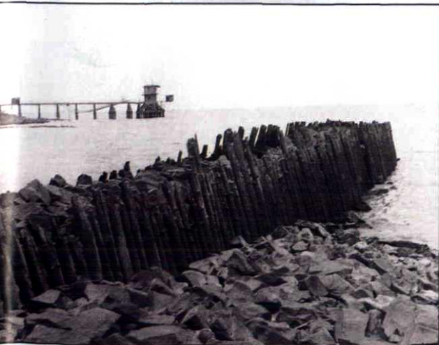
木桩砖石护滩工程遗迹 Historical remains of timber piles and masonries for beach protection
