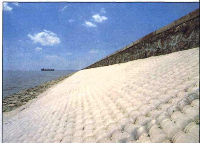
法布护坡 Revetment with fabric form
