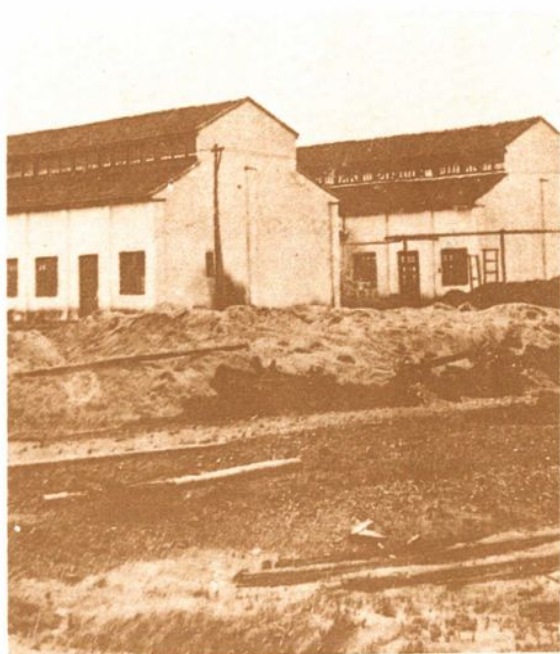
舊勝試驗性生產車間及鍋 爐間之遠眺
