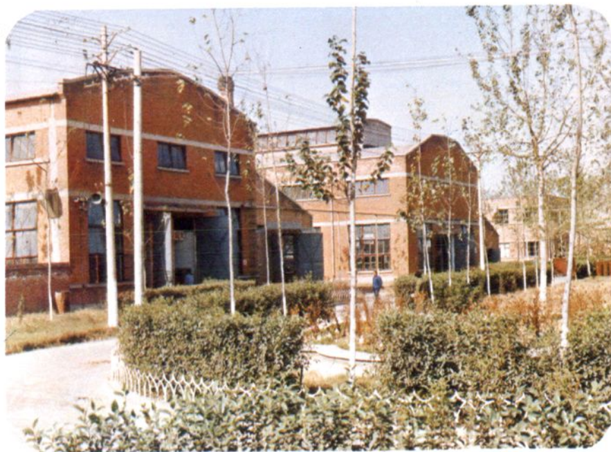
烤漆、锻压车间一角
