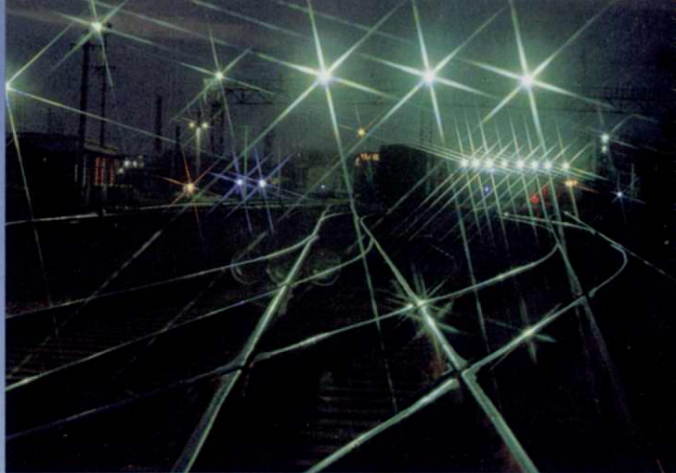
调车场 Truck dispatching field
