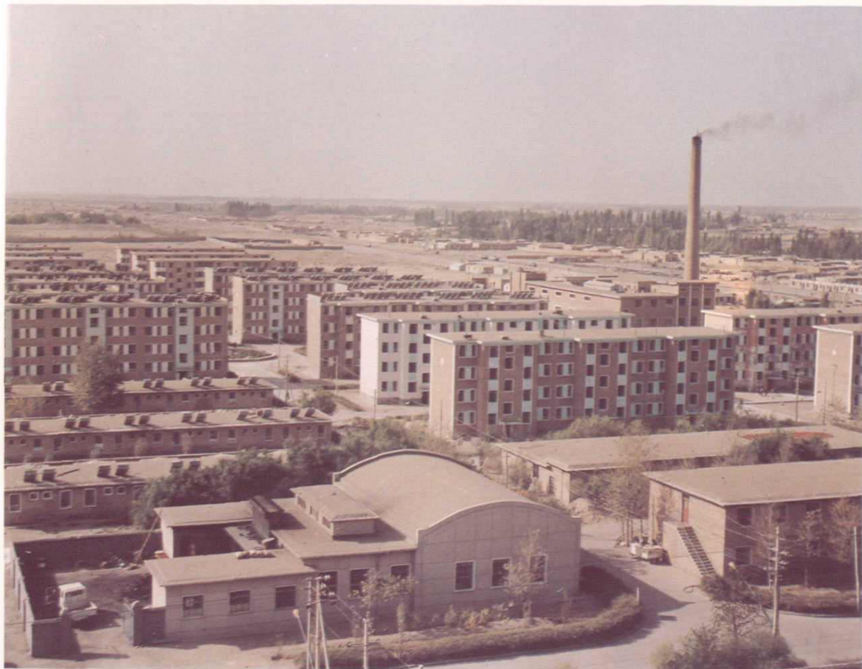
库尔勒市新城区物探三处基地 The No.3 department base of the Geophysical Bureau in xincheng area
