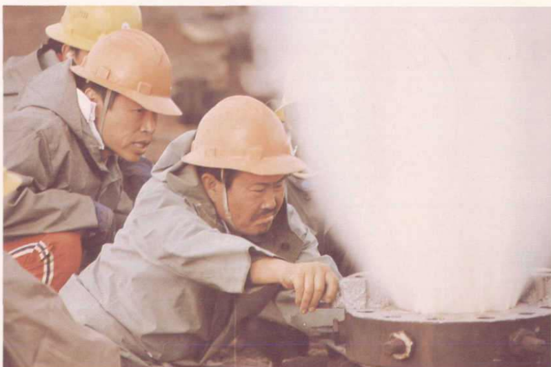
1990年甲乙双方共同治理轮南22井 井喷 Part A (TPEDB) stopping blowout of Lunnan No.22 well with Part B (the other unih).
