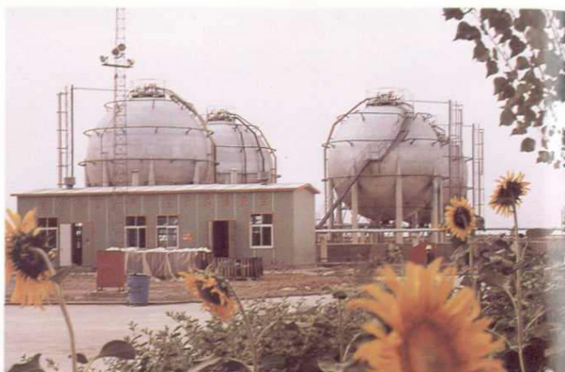
轮南油田轻烃站液氮储罐群 Liquid-nitrogen storage-tanks in lighter hydrocarbons station of Lunnan oilfield.
