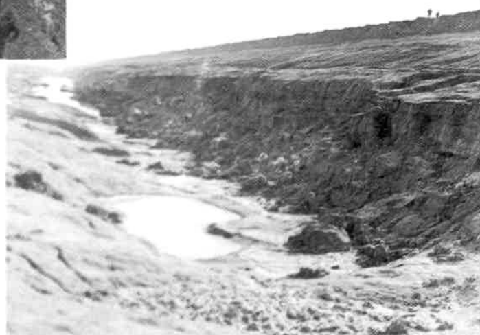
板桥水库大坝坡脚被冲毁
