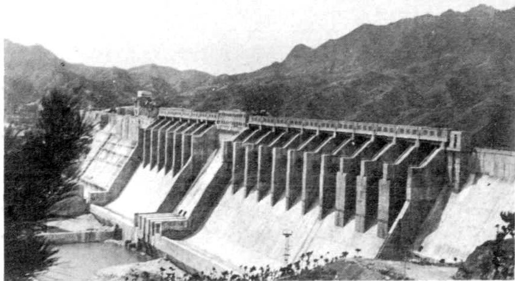
△潘家口水库大坝
