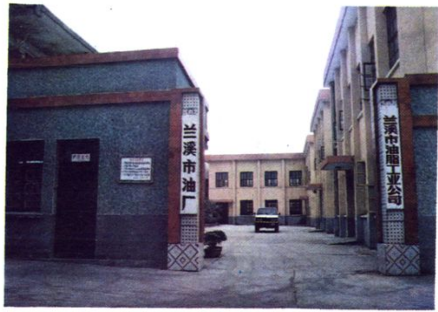
▶ 兰溪市油厂类可可脂车间
