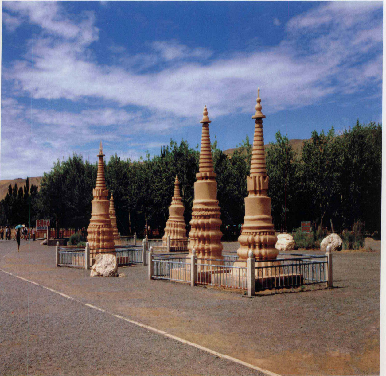
莫高窟的舍利塔 The newly repaired stupa of Mogaoku
