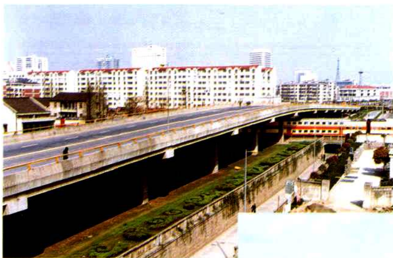
临平东湖立交桥
