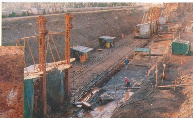
↑ 乌卡斯冲击钻造孔做大坝防渗墙
