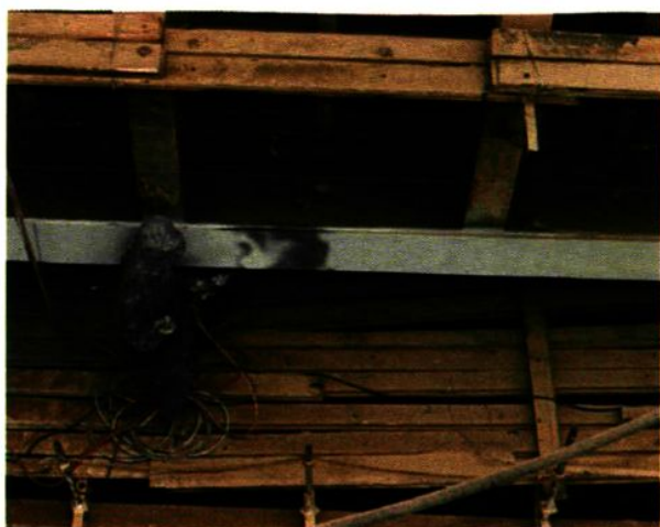
闸门除锈喷锌
