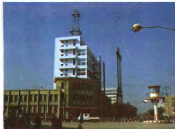
宿县地区邮电大楼
