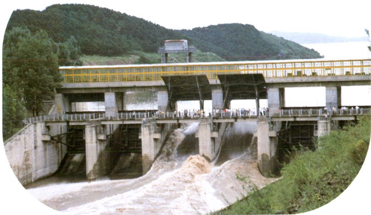
“95·7”水库溢洪道泄洪
